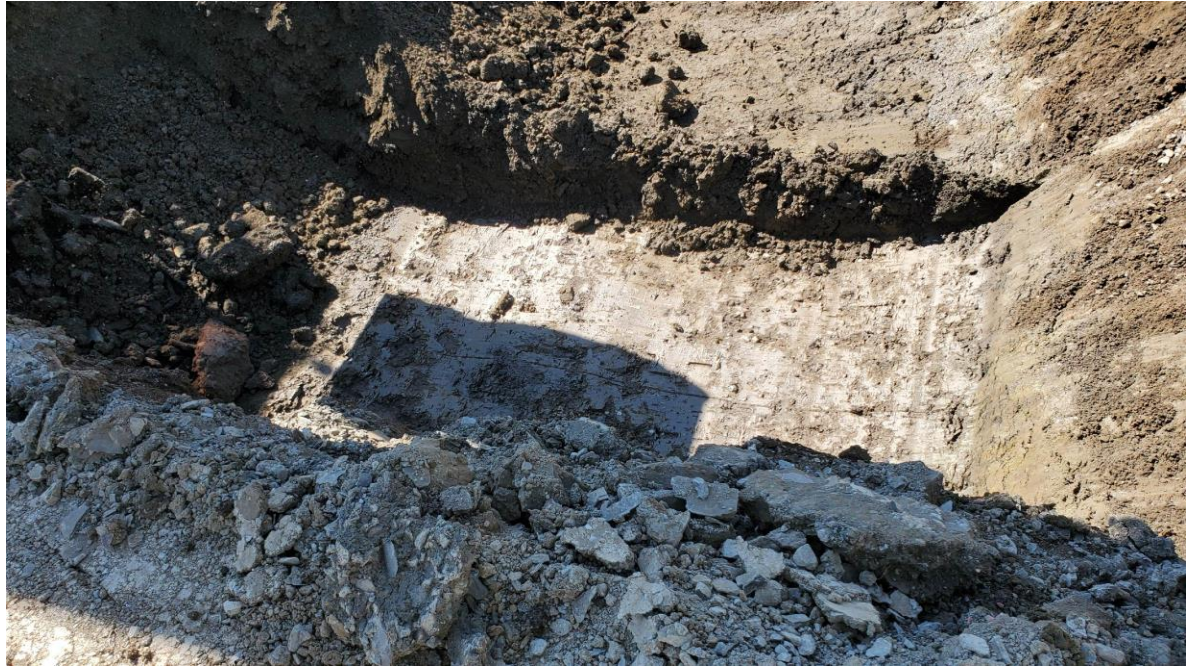
Photo 1. Exposed competent stiff CL subgrade soil.
